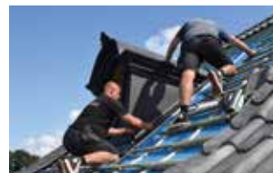
Installing the bull's eye on the wood structure
