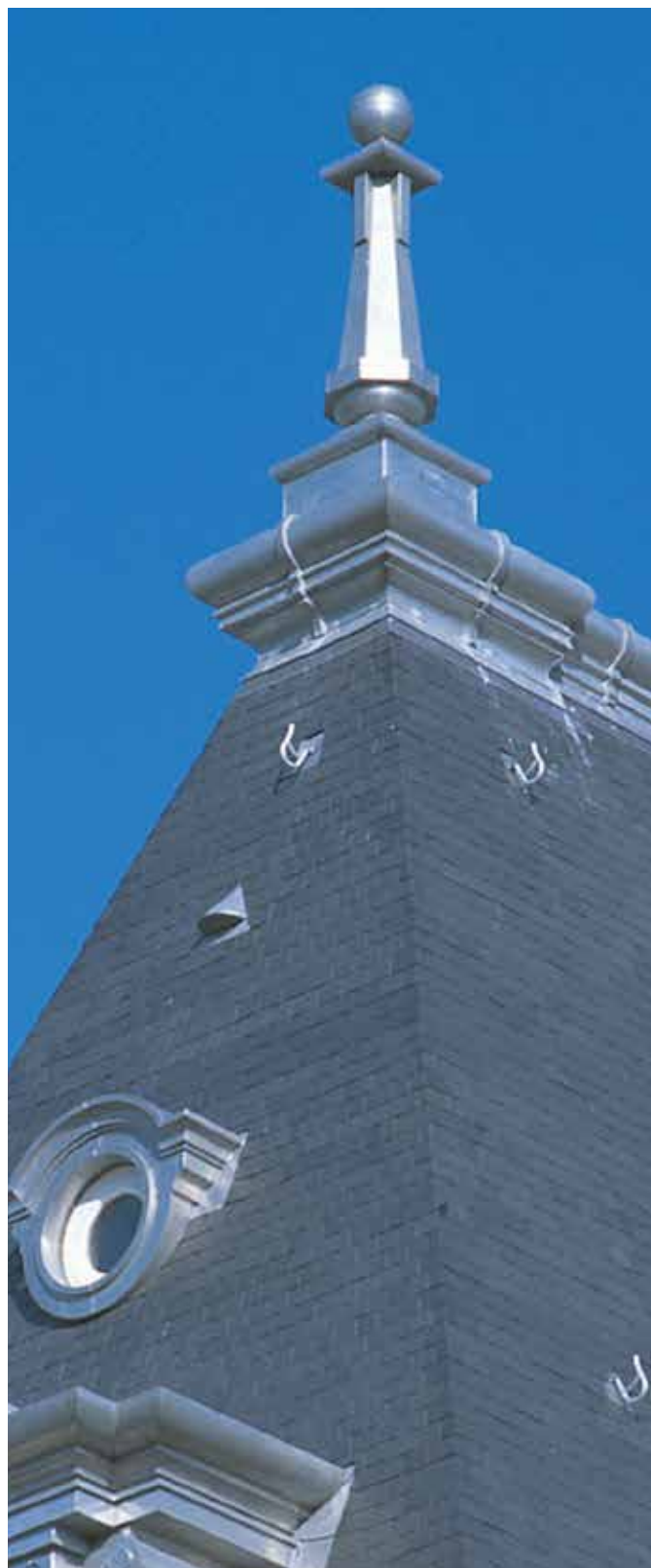
Town hall, Corbeil- Essonnes (France)*
