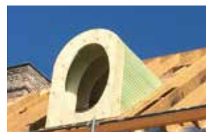
Installing the wood structure*
