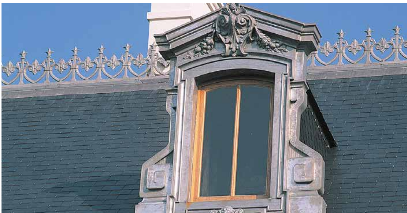
Town hall, Corbeil-en-Gatinais (France)*
