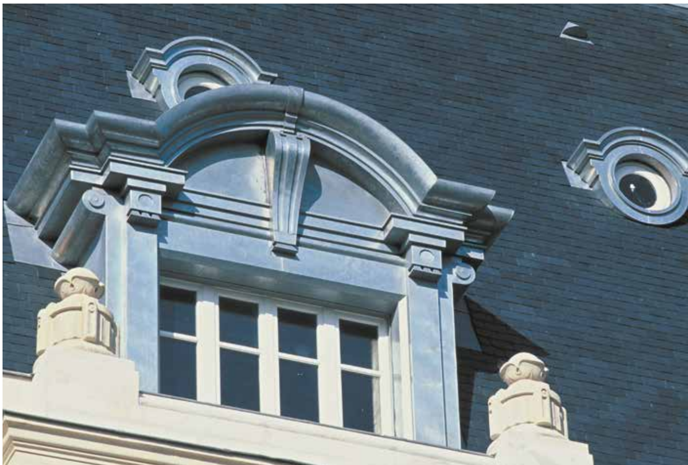
Town hall, Corbeil-Essonnes (France)*
