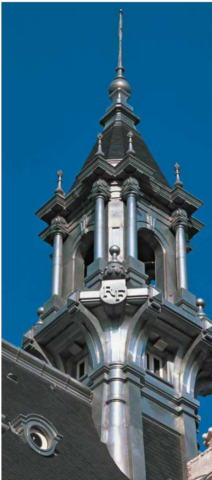
Town hall, Corbeil-Essonnes (France)
